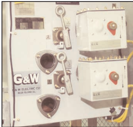
▲ Front mounted actuator with stored energy mechanism on an SF6 switch.
