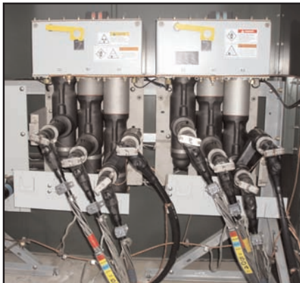
▲ G&W Trident solid dielectric switch with integral magnetic actuator.
